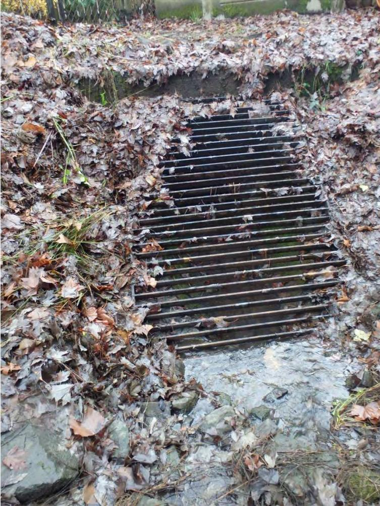
Photo 7 36-inch culvert under SW Willow Creek Drive
