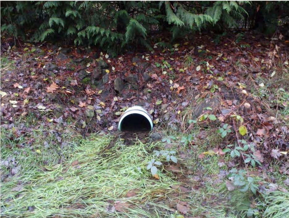
**Photo 6 Partly submerged 18-inch CCP contributing culvert**
