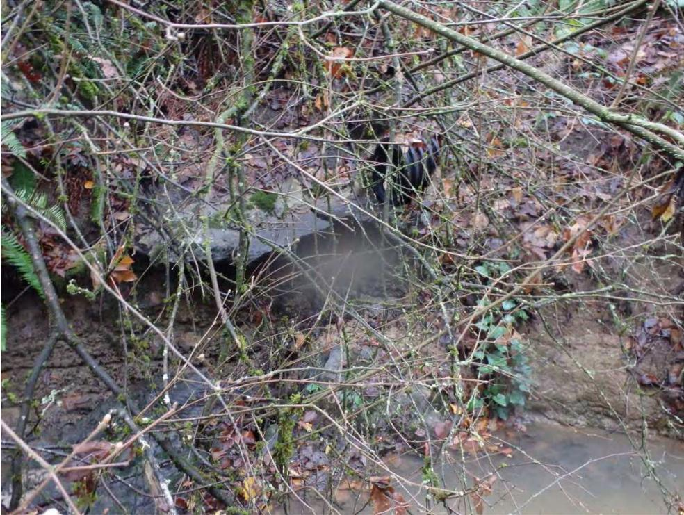
**Photo 16 Perched Culvert on Right Bank**
