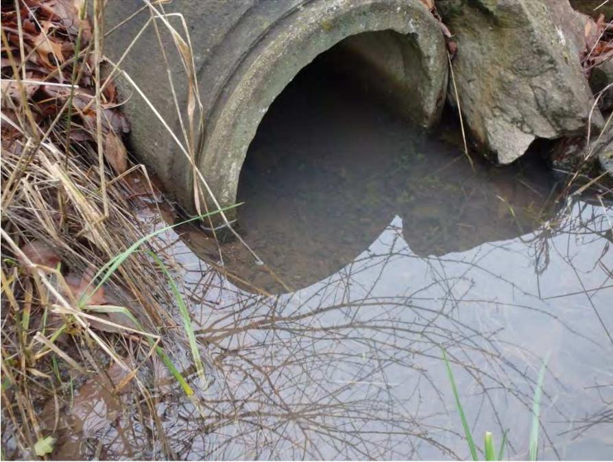
**Photo 3 Downstream of culvert with gravel accumulation**
