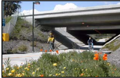
Type 4 Grade-Separated Undercrossing
