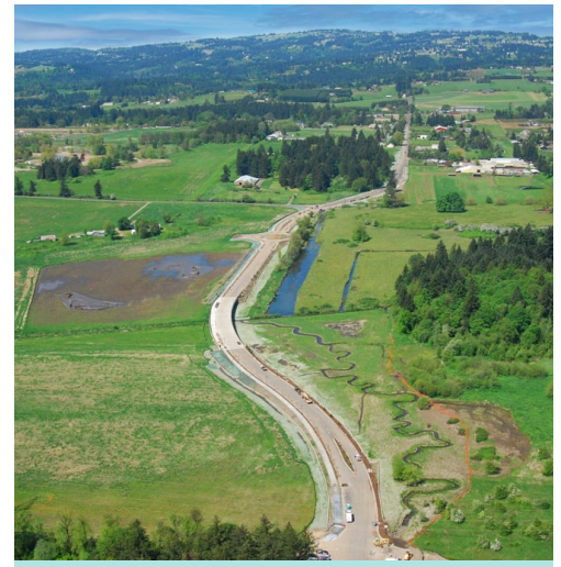
Boeckman Road Construction (2008)
