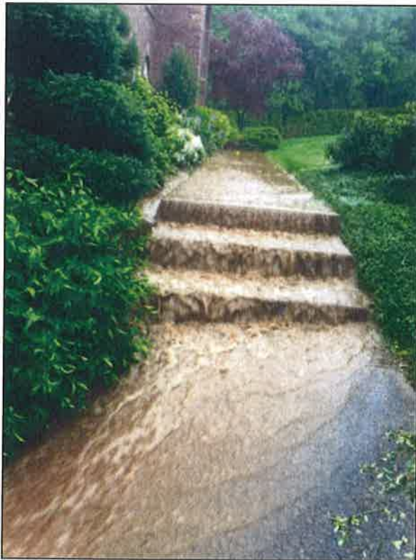
Photo A6. The front walkway steps drain into the lower driveway and garage area.
