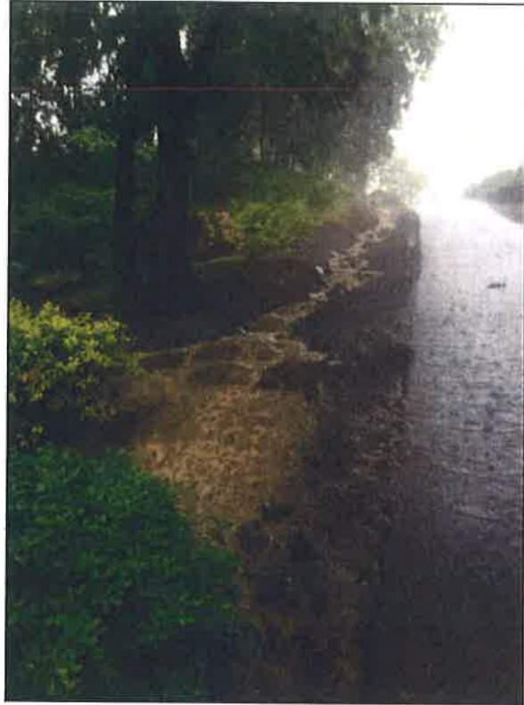
Photo A3. The junction for the channel and driveway pipe are overwhelmed and flood waters drain into the front yard toward the house.
