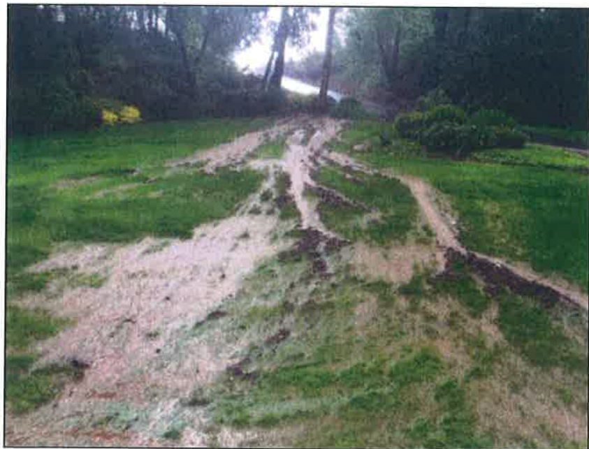
Photo A4. Flooding storm water ultimately found its way into the lower driveway area.
