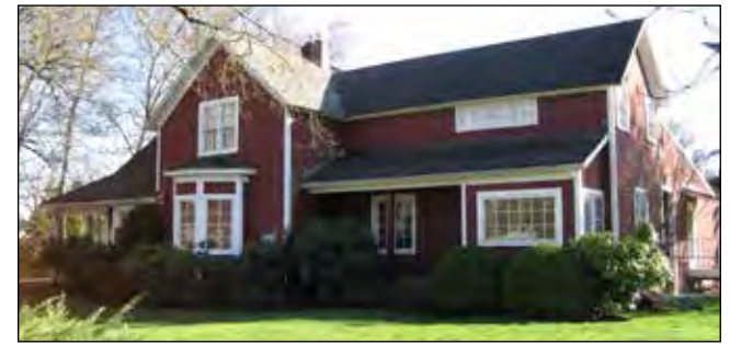
The home previously occupied by the Northwest Montessori School is approved for light-duty office use.
