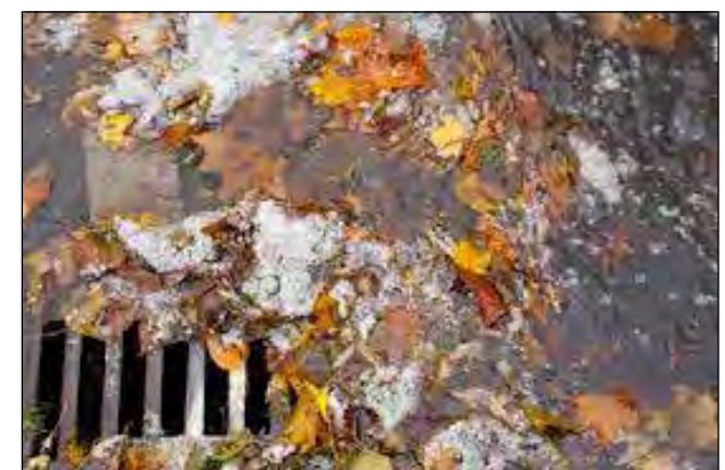
Community members are encouraged to remove leaves and other debris from storm drains to prevent localized flooding.
