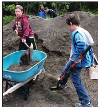
WERK Day volunteers shoveling gravel to be laid on the path to Memorial parks Off Leash Dog Area.
