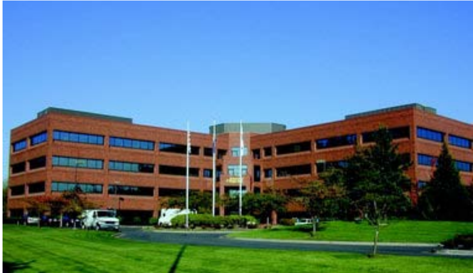
Figure 30 Mentor Graphics Headquarters Office Building in Wilsonville.
