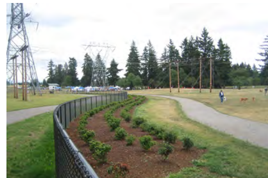
Park integrated with power line easement
