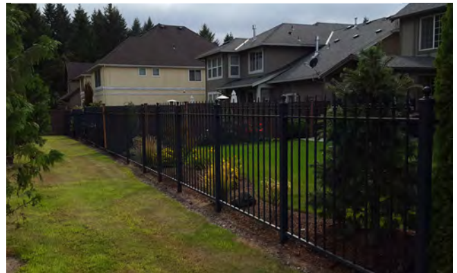
Figure 12. Examples of Creekside Treatment
