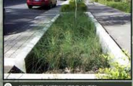
10 STREET SIDE STORMWATER PLANTER
