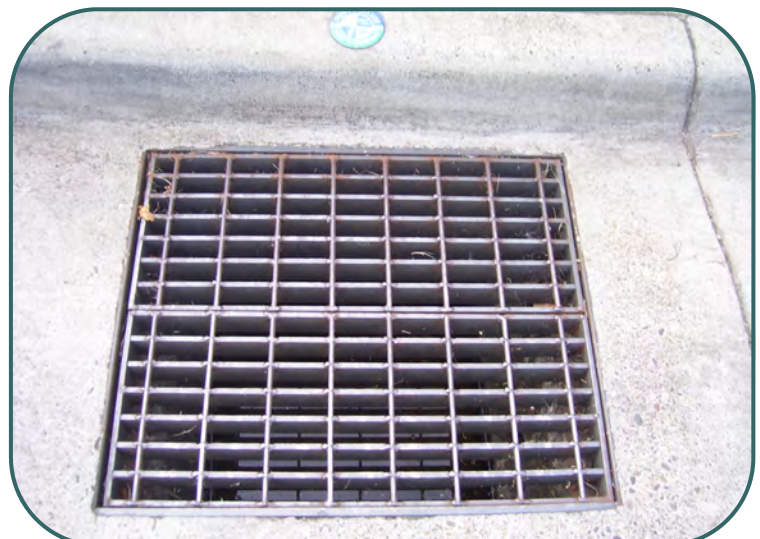
Well maintained catch basin
