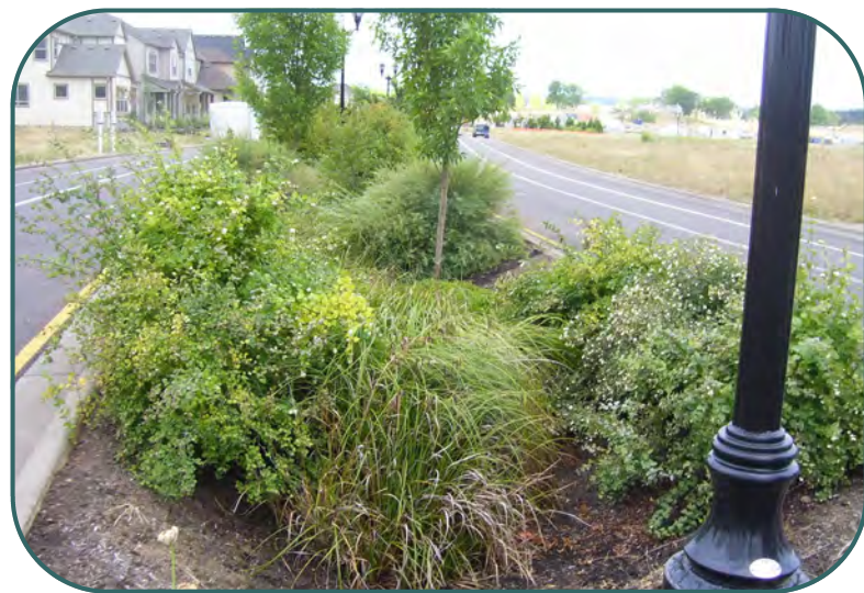
Well maintained swale
