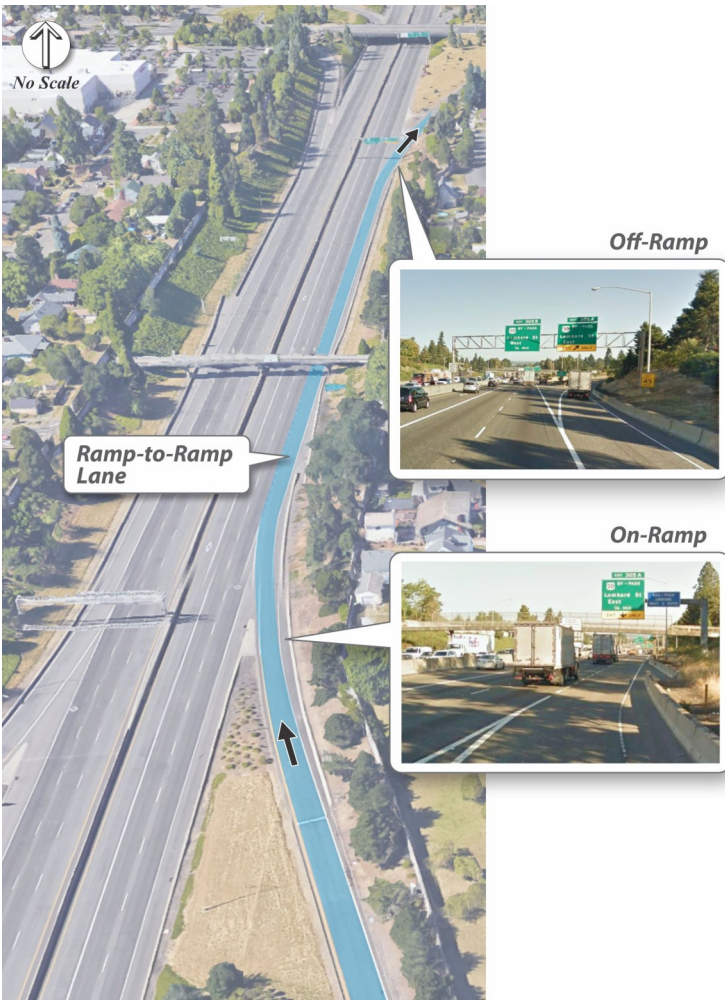
FIGURE 10. A ramp-to-ramp lane on I-5 NB between the N Rosa Parks Way on-ramp (304) and the N Lombard St East off-ramp (305A). This ramp to ramp lane is 0.2 miles long, comparable to the distance between the Charbonneau and Canby-Hubbard off-ramps.
