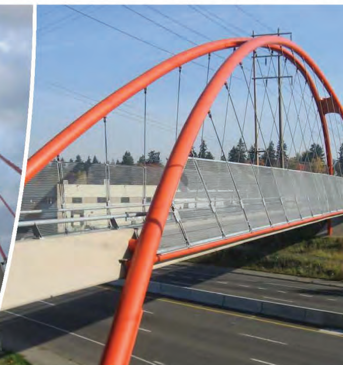
Springwater Trail Bridge
