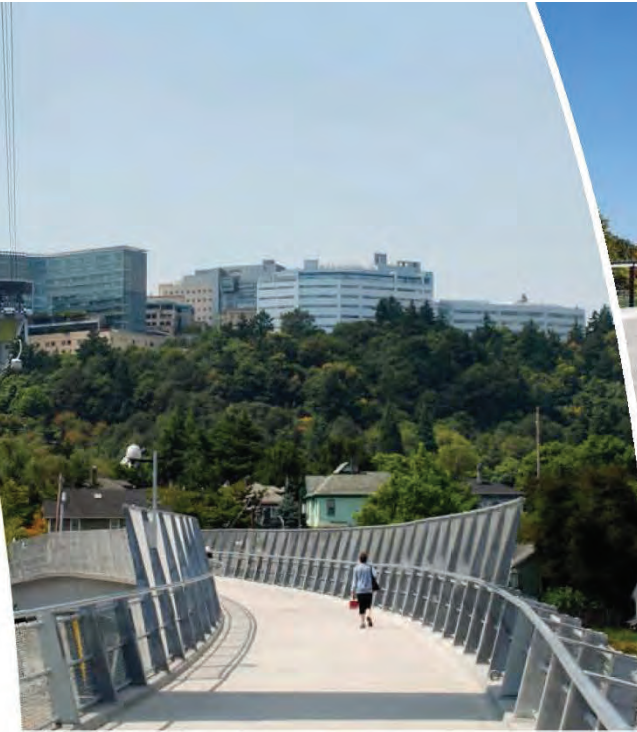
Gibbs Street Bridge
