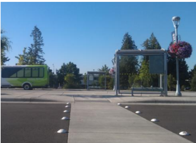
Curb ramps with gradual slopes and large transit pads at the SMART Central transit center can accommodate users in wheel chairs or with other special needs.
