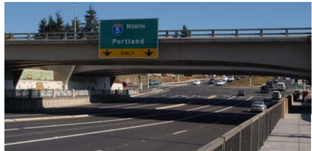
Looking east to the I-5/Wilsonville Road interchange.
