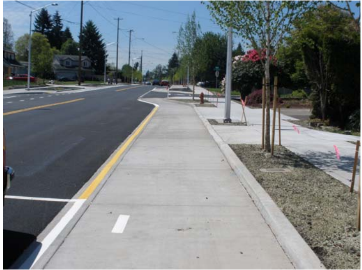
One-Way Cycle Track on Cully Boulevard in Northeast Portland. Cycle tracks are typically protected from motor vehicle traffic by parked cars, raised curbs, or other physical buffers.
