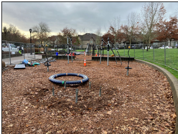
Sofia Playground Removal.
