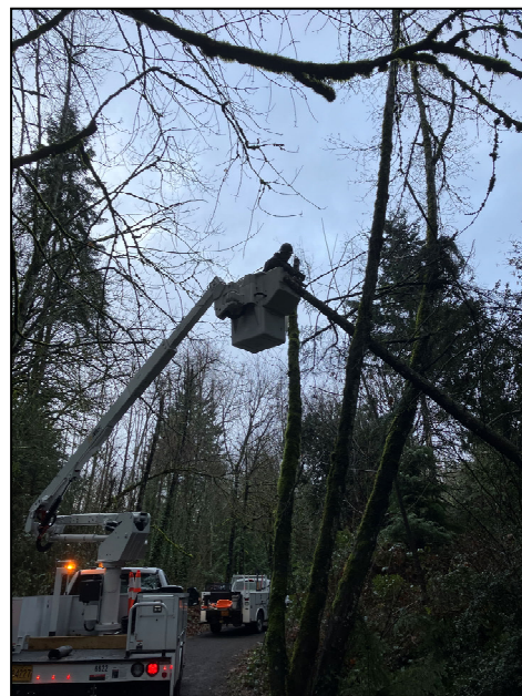
Hazard Tree Removal.
