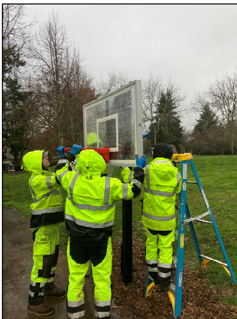
Basketball Hoop Install.
