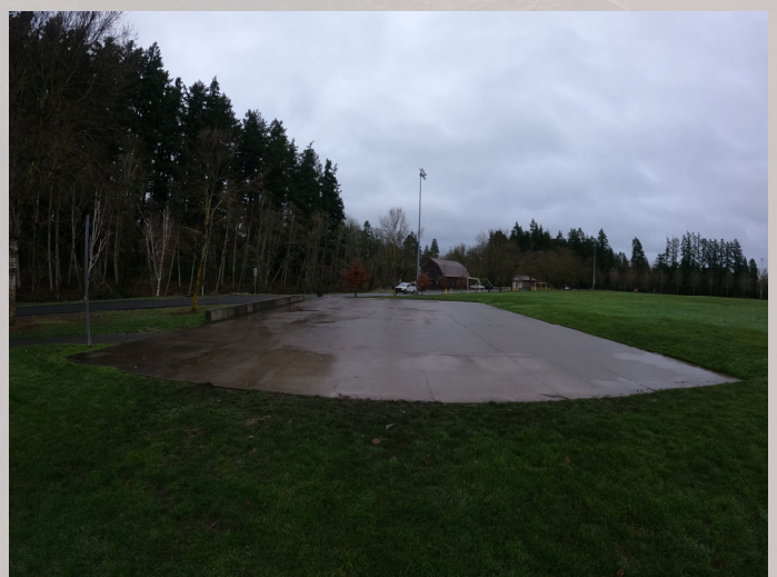
Remaining Concrete Pad
