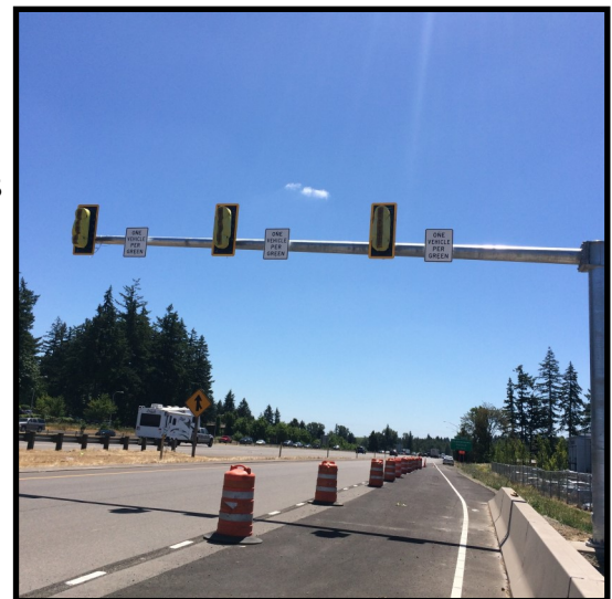
Coming Soon—New Ramp Meters
