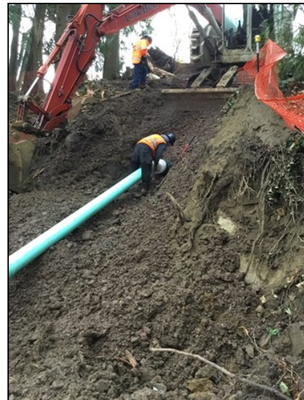
Slope and outfall repair
