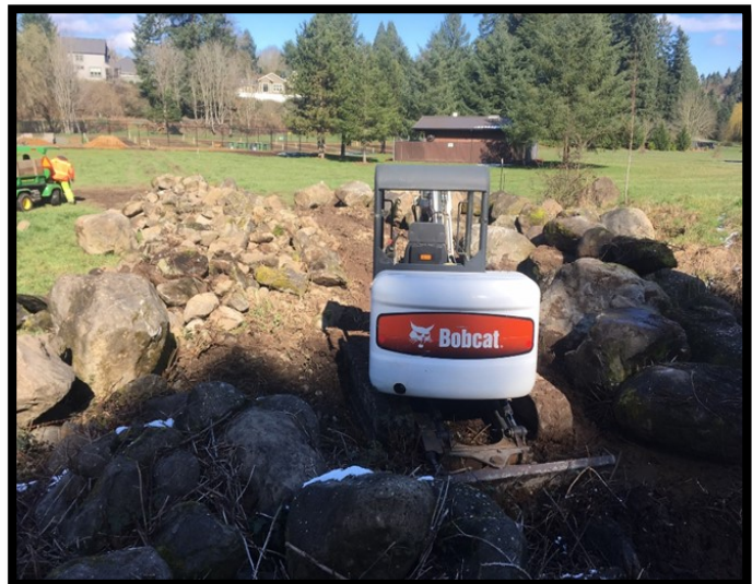
Began preparations for expanded Community Garden Parking Lot
