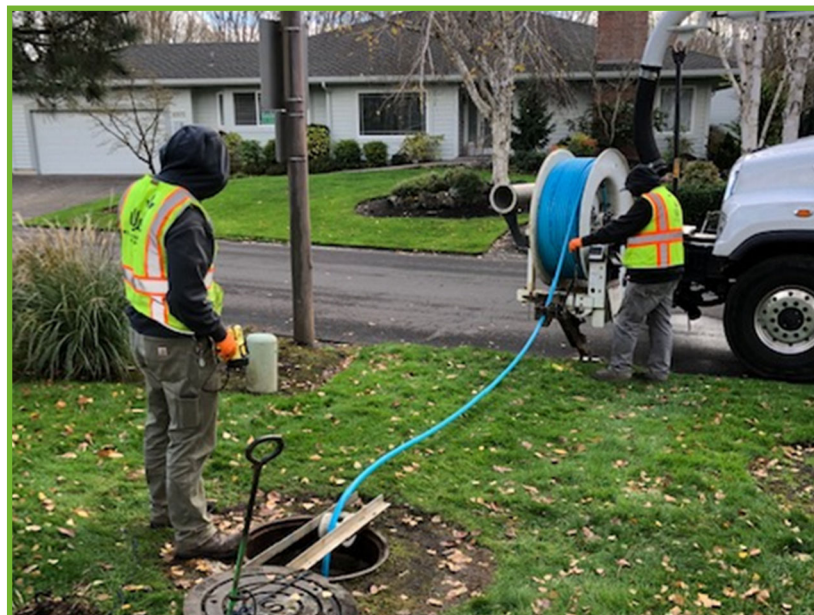
Jetting the line to remove debris
