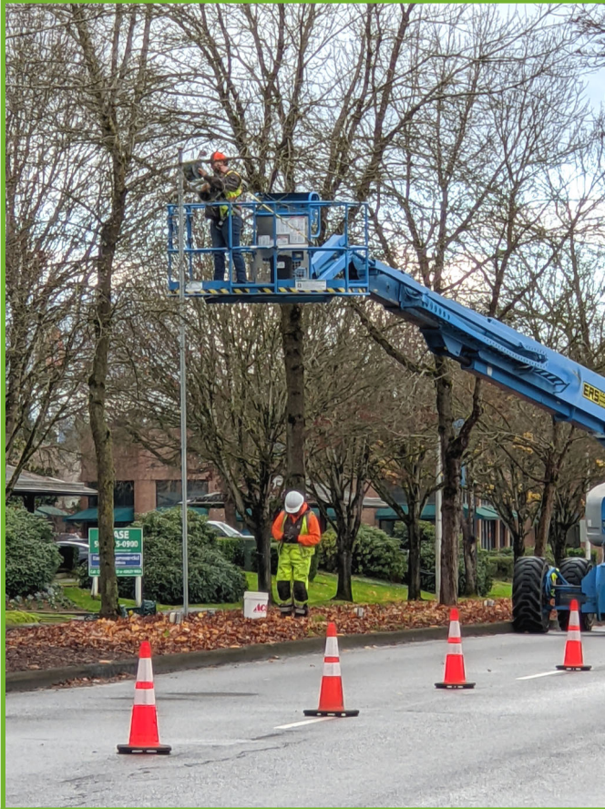
Adding lights to the trees in the median
