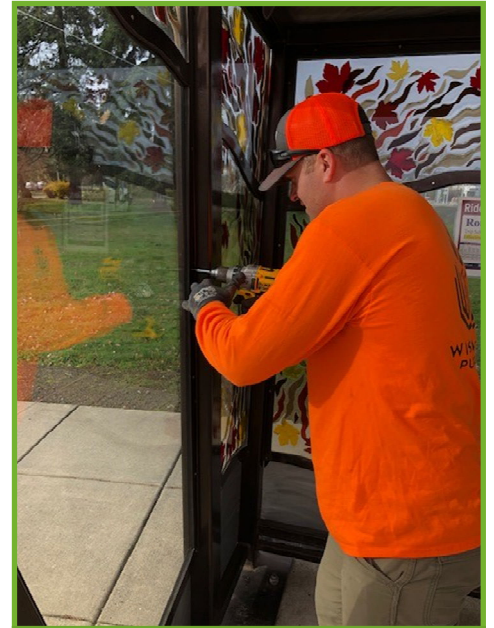
Trevor removing glass panels
