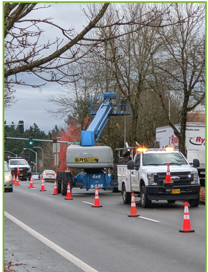
Working safely in the roadway
