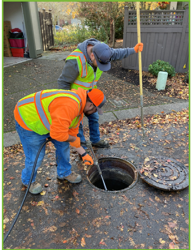
Jetting through the obstruction
