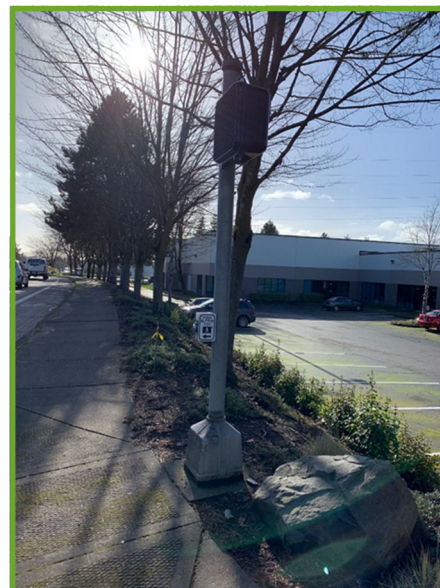
New crosswalk signal
