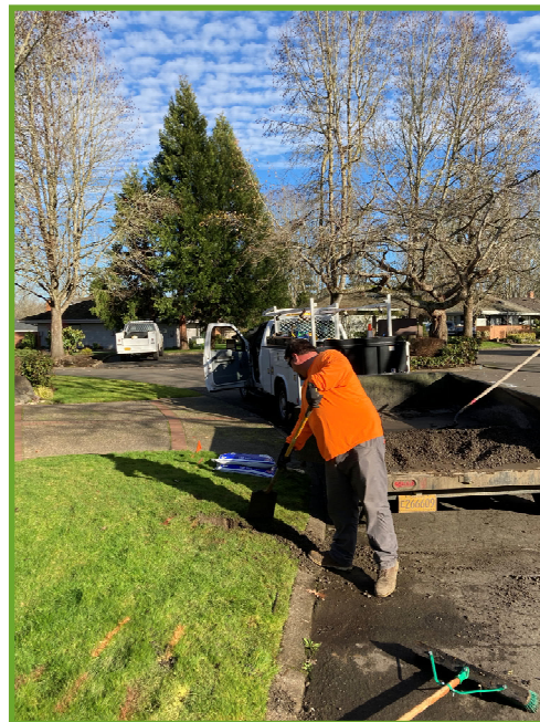
Backfilling the pothole
