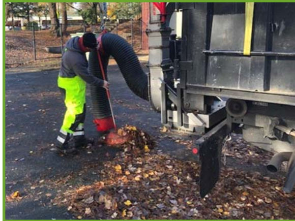
Custom vacuum trailer at work
