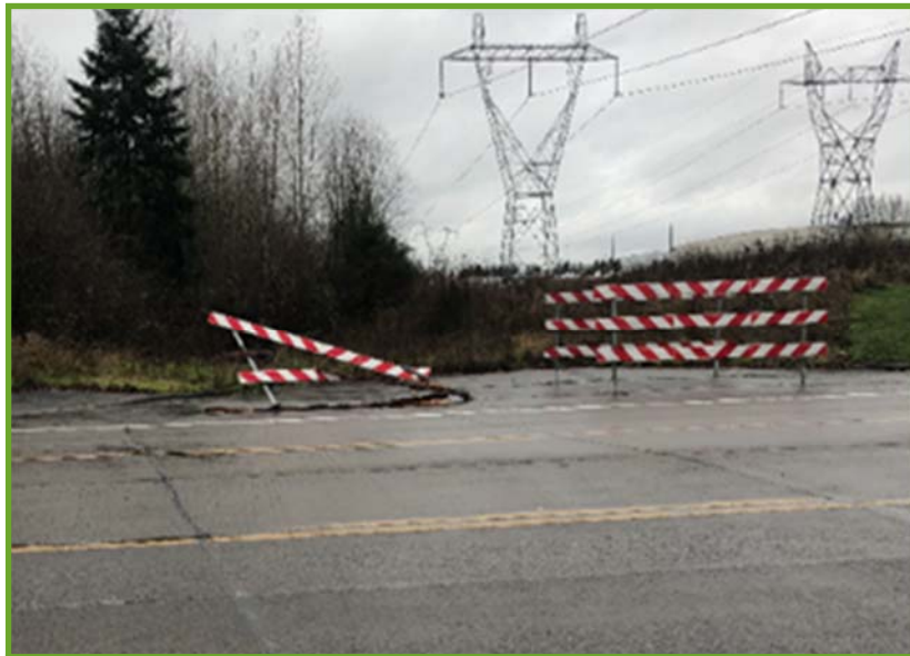
Severely damaged barricade
