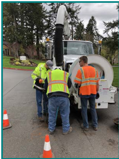
Left: Acting Water Tech Sam Kinnaman receives cross training from Sewer crew members Paul Havens and Paul Walker on how to jet sewer lines.
