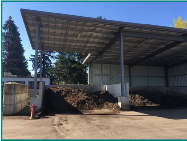
Decant facility for Vector & catch basin materials.
