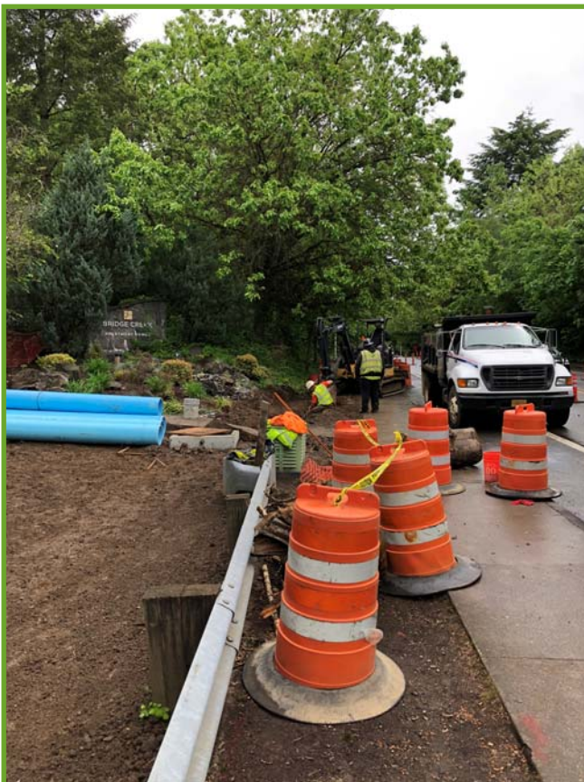
Project work site along Wilsonville Road.
