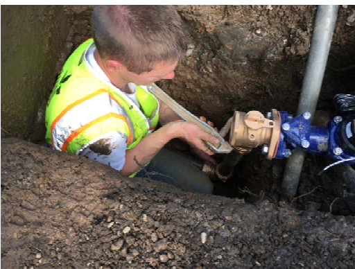
Tightening pipe fittings
