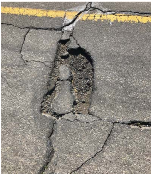
Pothole before being fixed
