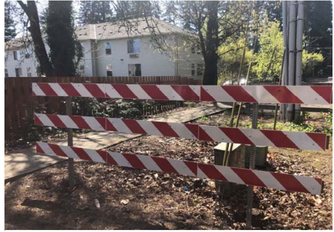
Replacement barricade with steel posts
