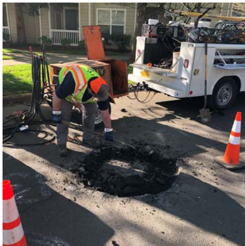
Preparing foundation for casting ring installation
