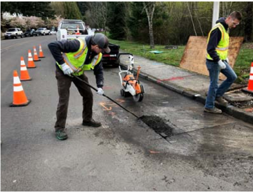
Removing asphalt pavement
