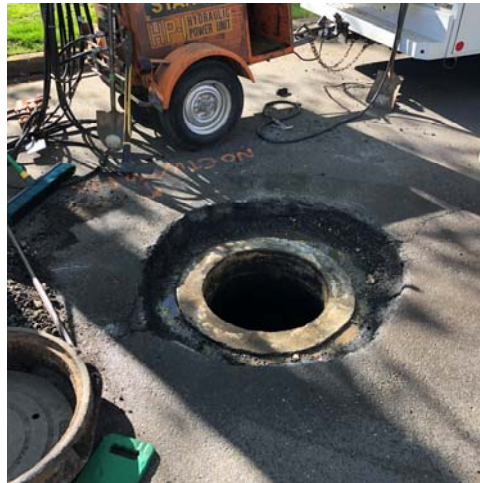
Removing casting ring foundation
