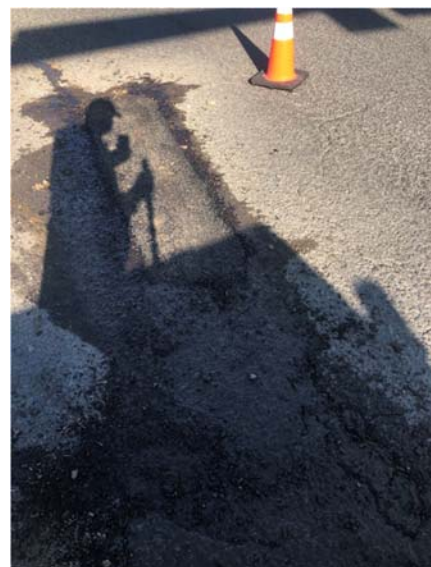
Pothole after repair
