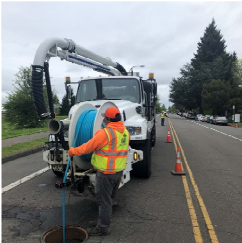
Cleaning sewer main
