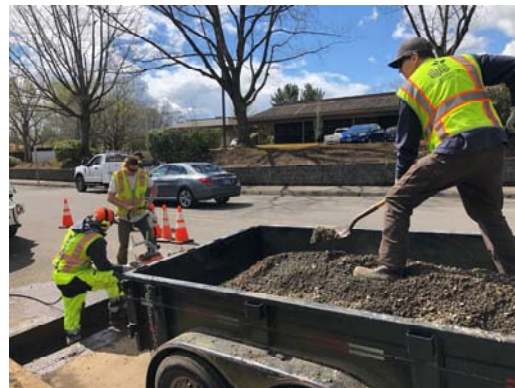
Backfilling excavation
