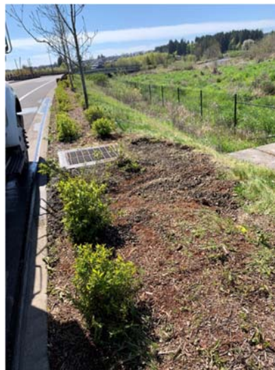
Restoration of sink hole area
