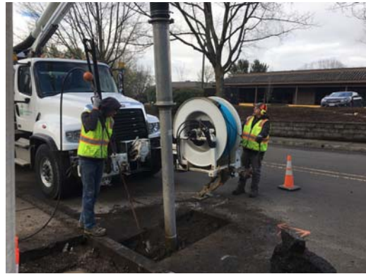
Excavating hole with vacuum truck
