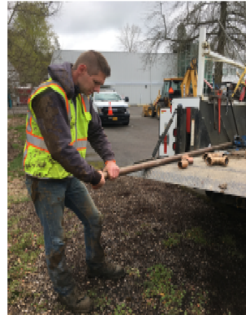
Preparing new copper pipe
